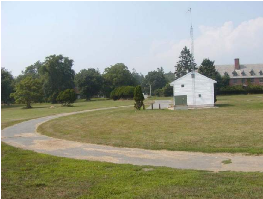
Photo 3-11. Municipal wastewater pump station
