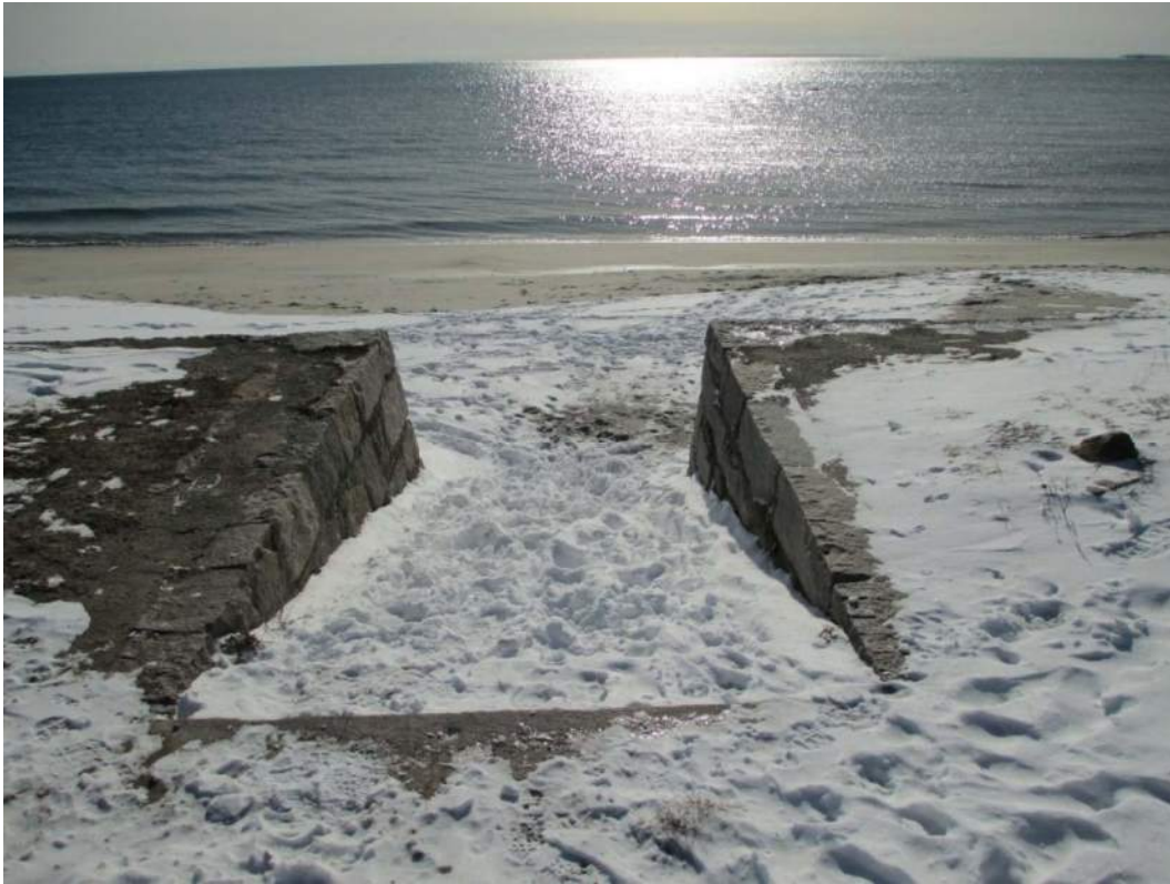
Photo 3-16. Stairway in seawall leading down to beach
