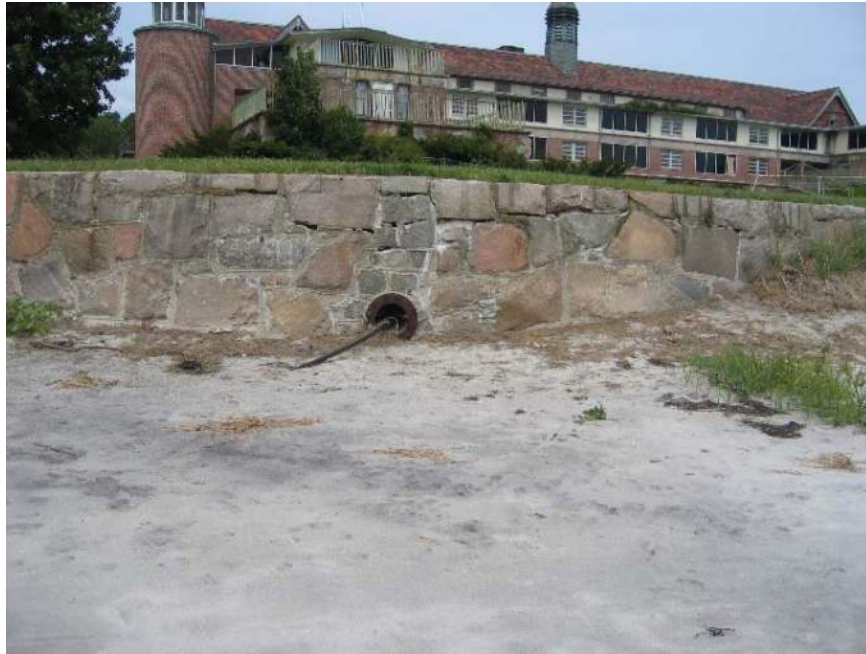
Photo 3-3. Culverted stream outlet to central pocket beach at base of seawall
