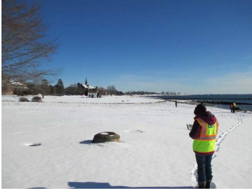
Photo 3-12. Elevated sewer manhole along easement
