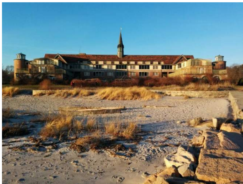
Photo 3-2. Pocket beach, seawall and beach grass in front of Main Hospital
