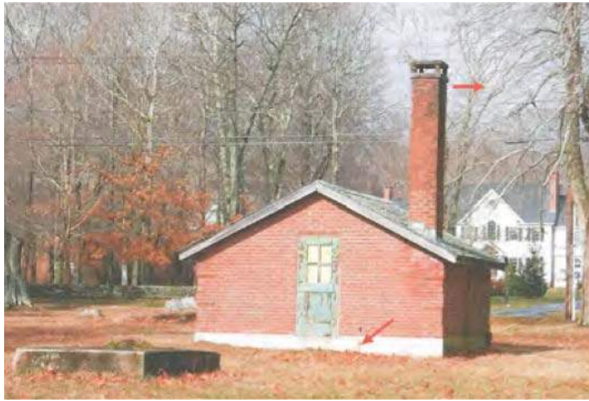
Photo 3-26. Old Pump House
