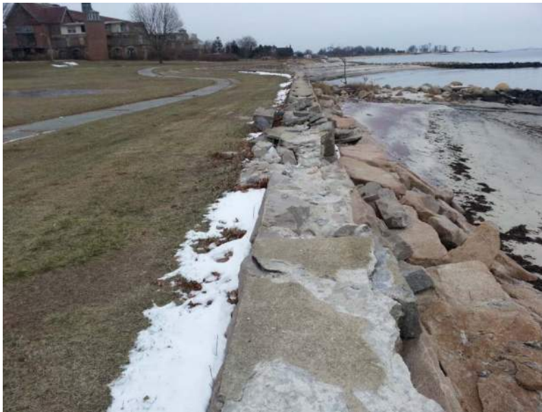
Photo 3-9. Easterly view along seawall at central cove
