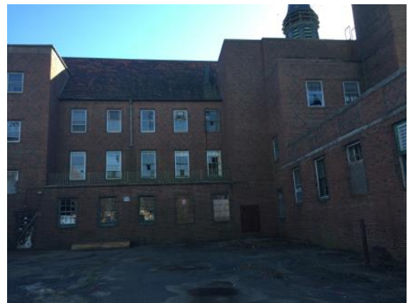
Main Hospital Building
