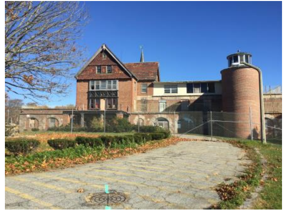
Main Hospital Building
