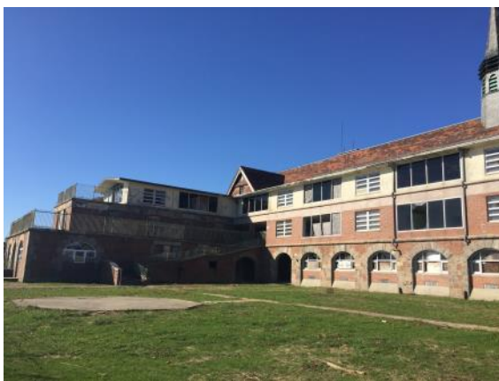
Main Hospital Building
