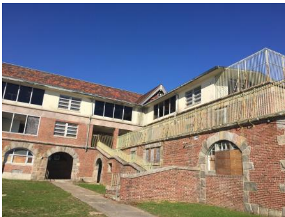
Main Hospital Building
