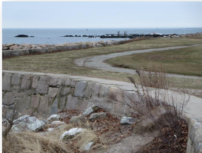
Seaside State Park - Seawall
